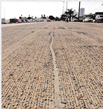
if possible, wait several days to a week to pave the new overlay once the sealant has been applied. This will allow the material settle properly.
