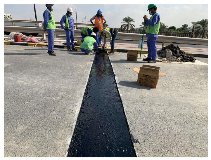
The final top layer of the Matrix 502 Mixture is then installed to approximately 6-12mm above the existing surface to allow for compaction. Compacted Joint is then allowed to cool until the surface temperature reach atmospheric temperature.
